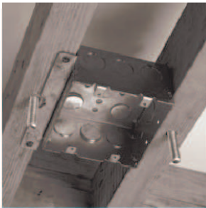
4" junction box and 5-3/4" bolt circle Figure A
