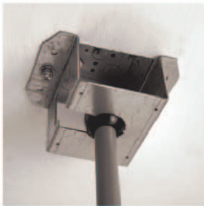
Hang straight bracket and pendant Figure B
